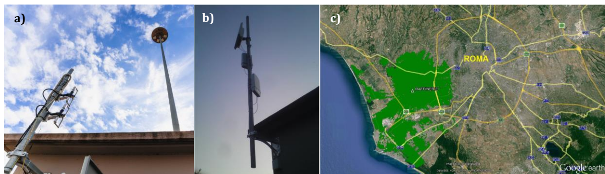
Figure 4: a) HiperLAN and Tetra equipment installed on a secondary substation of the pilot project; b) detail of the HiperLAN antenna; c) TETRA coverage of the project area
